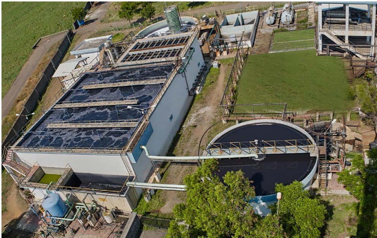
1.5 MLD textile effluent treatment plant at Tessitura Monti (Kolhapur) featuring AAA™ technology. Project execution by A.T.E. Envirotech
