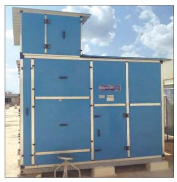
15,000 CFM HMX-Ambiator installed at Himalaya's Bangalore plant
